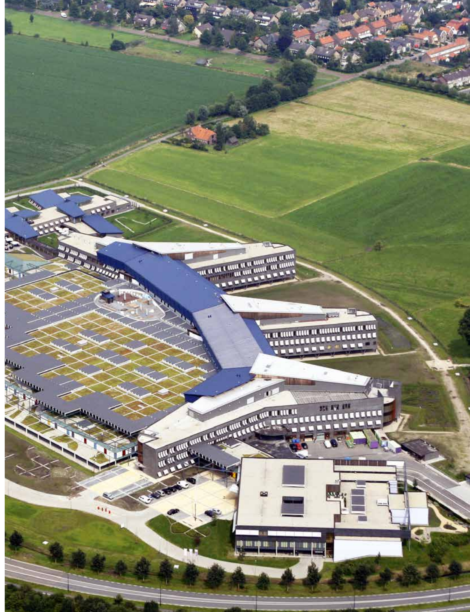
Deventer Hospital, Deventer, the Netherlands (example of a sustainable design)
